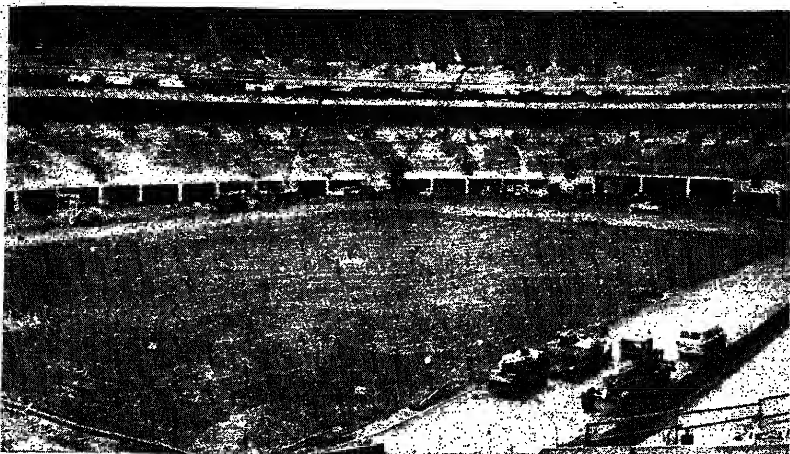
This is how the Olympic Stadium in Montreal looked Friday. To finish construction in time, there are 2,000 workers by day and 1,500 by night.
